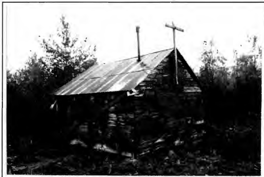
Figure 71. The NADC Pump House, 1993. The view is looking northwest.
